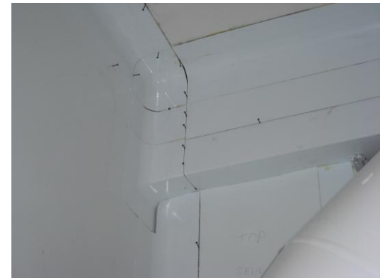
Preformed corners adhered to fiber-reinforced wallboard
