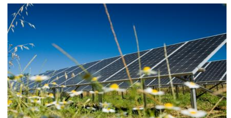
Solar and Green Waste Treatment
